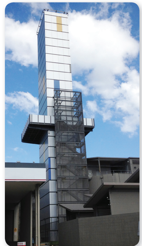
Marsden Street Ventilation Stack, Artarmon, Lane Cove Tunnel.
